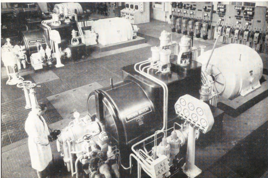
New electric power station, Pyrmont Refinery. The turbines are driven by high pressure steam from the boiler station. Low pressure exhaust steam from the turbines is used in the refinery. At left, Mr C. F. Rigby, chief engineer, Pyrmont Refinery.
