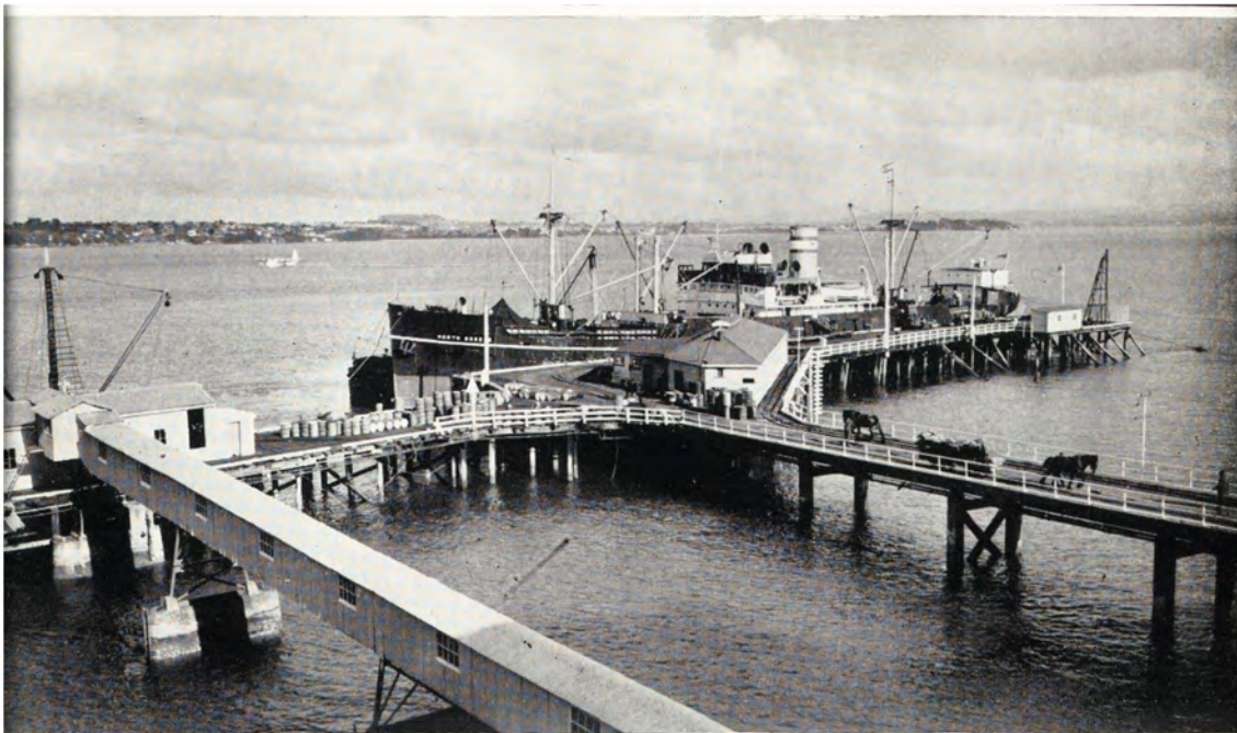
Overseas ship discharging raw sugar at Auckland refinery, New Zealand.
