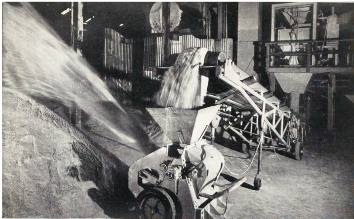
A mechanical thrower piling raw sugar from the mill process on the floor of the bulk store at the company's Harwood Mill on the Clarence River, N.S.W.
