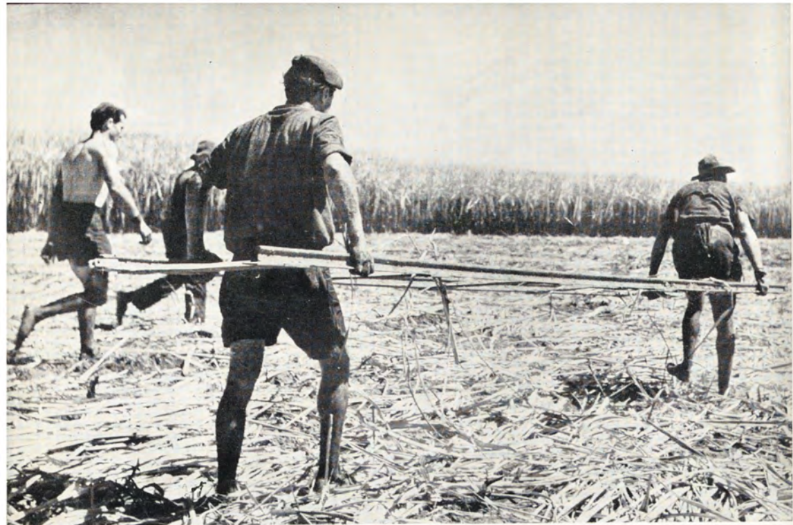
Laying portable line in cane field.
