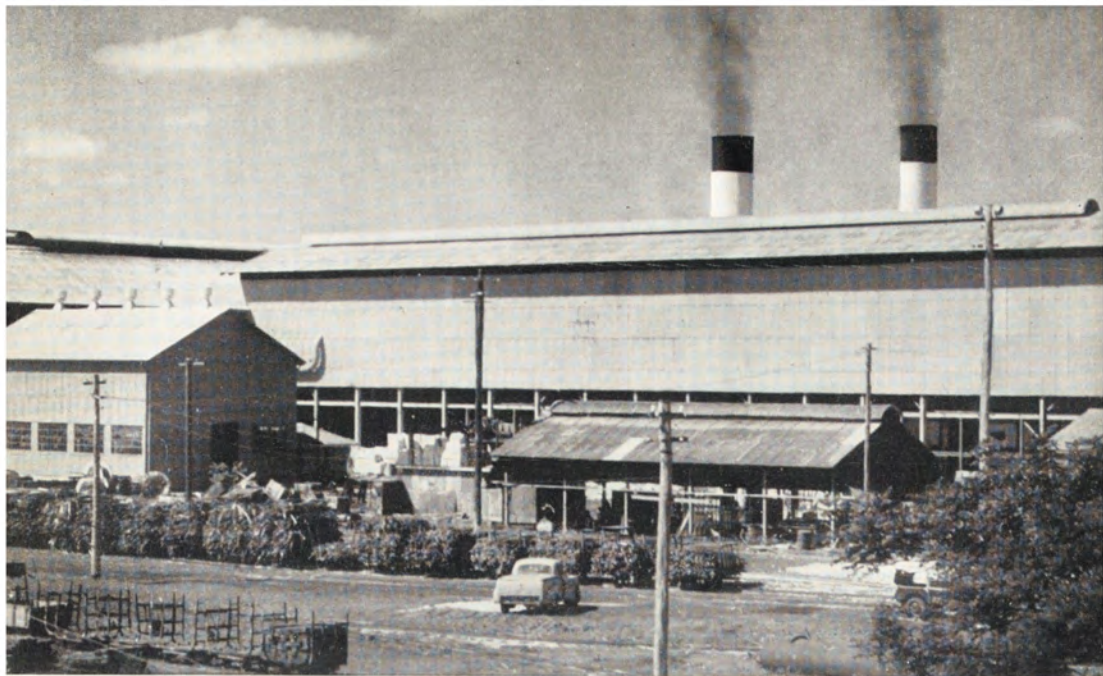
Power house and boiler station at the company's Victoria Mill, Queensland.
