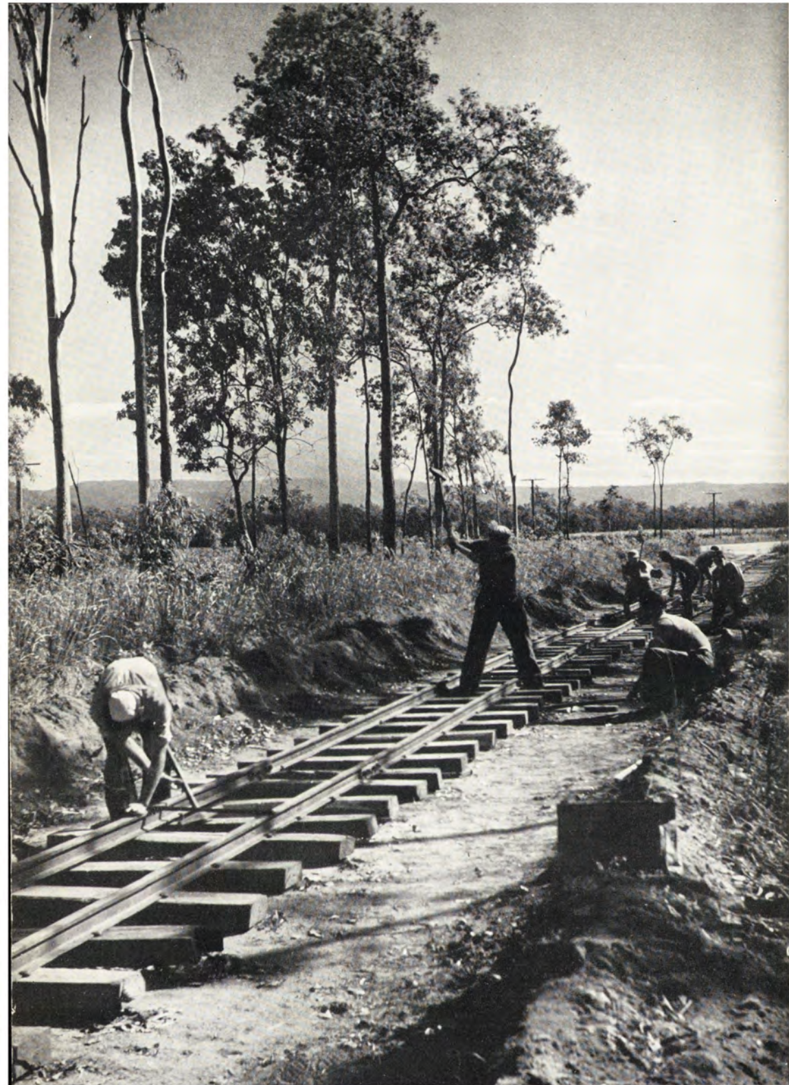
Laying a new light railway line to bring harvested cane from the recently opened-up Abergowrie district on the Herbert River, North Queensland.
