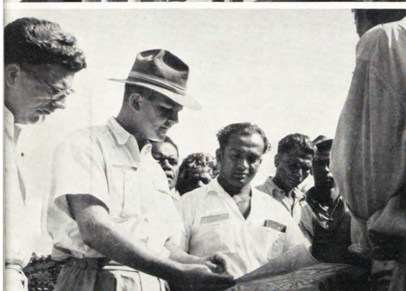
Instructing workmen, Lautoka.
