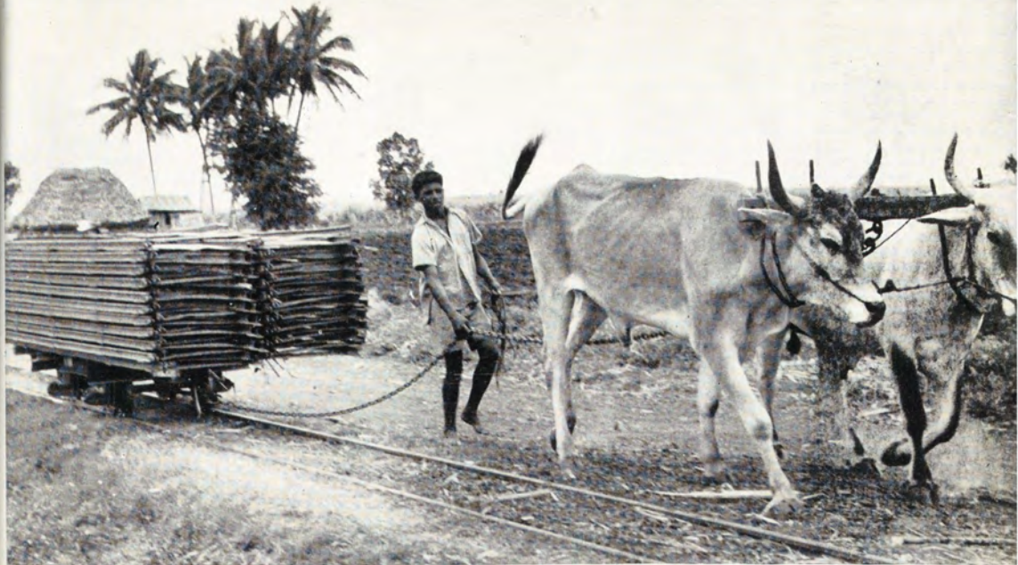
Hauling lengths of portable line to the field. Fiji official photograph.
