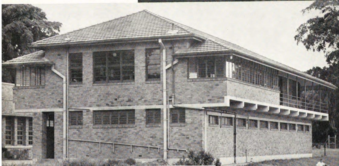
Amenities block, New Farm Refinery, Brisbane.
