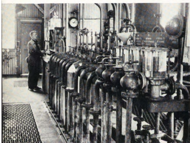
Left: Control panel and flow gauges, continuous esterification plant.
