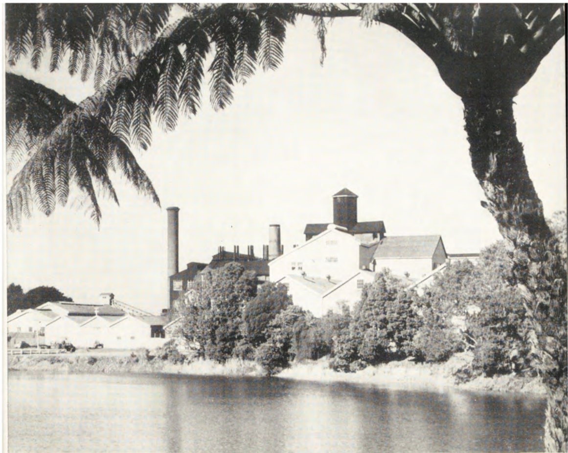
Chelsea Refinery, Auckland, New Zealand.
