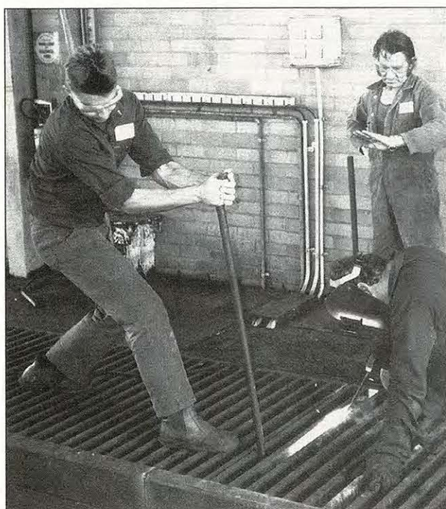
■ Engineers left to right: Eric Gourley, Graham (Sandy) Whyte and Doug Forbes converting the rail receiving area for road use in 1989.
