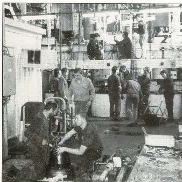
■ The maintenance team at work on the "Heart and Lung Transplant" at the Affination Station.
