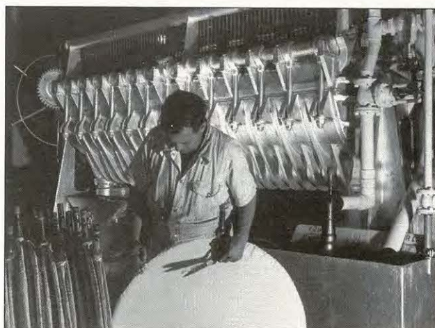
■ Davie Man repairing the filter cloths by hand. Filter station in background.
