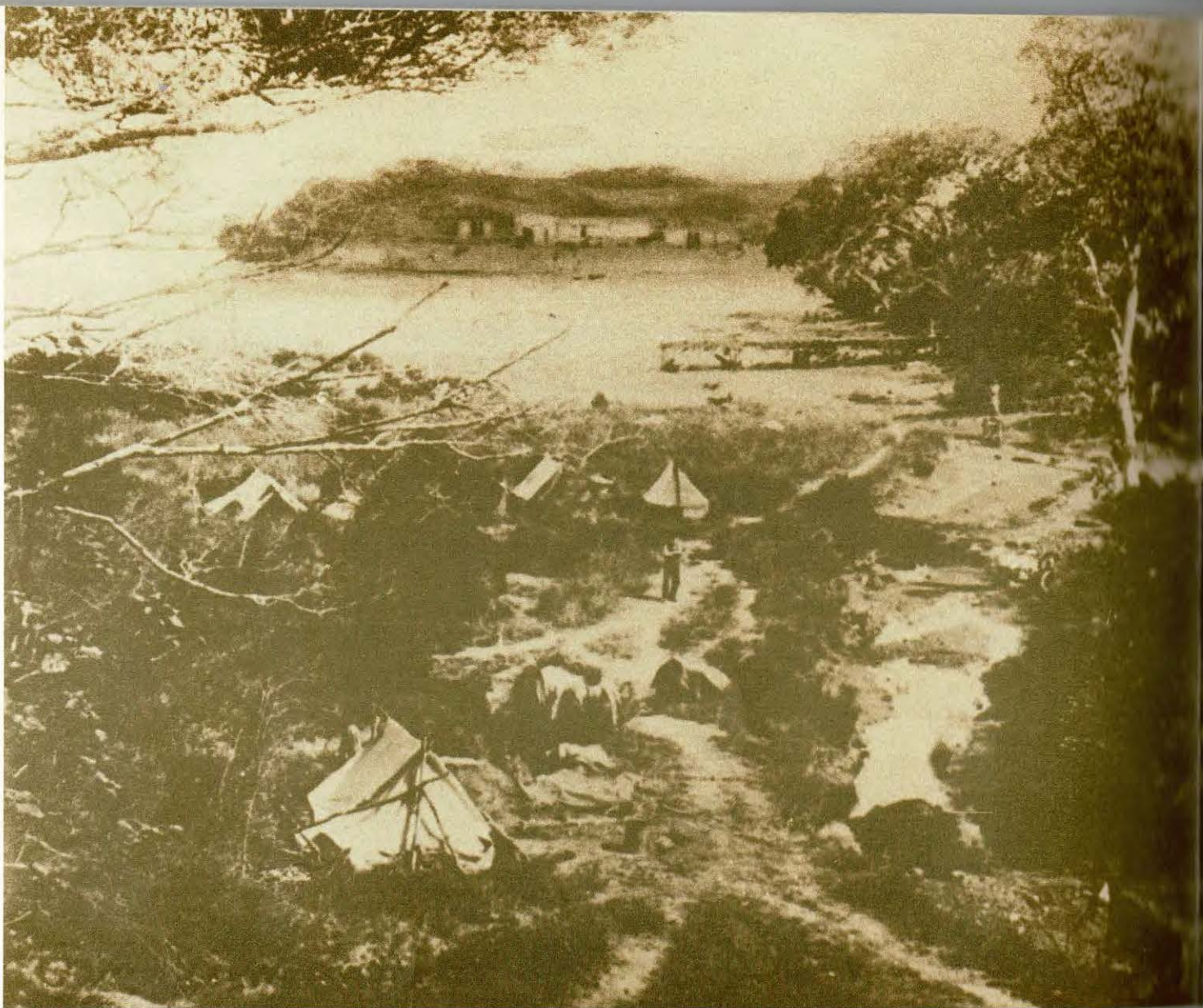
The Chelsea site, 1883. Behind the tents of the shanty town lies the half-built refinery.
