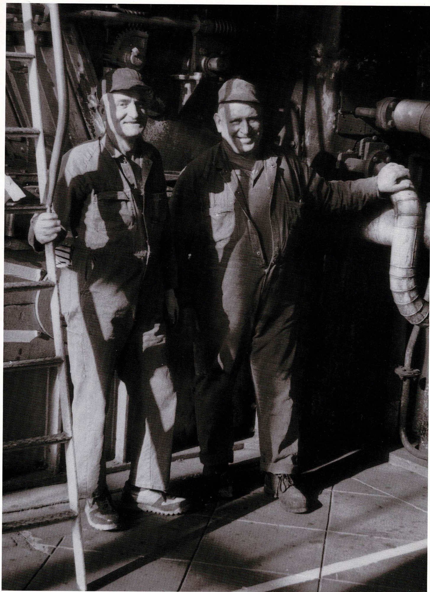
George Belivanis and Domenic Melacrinis in the Boiler Station
