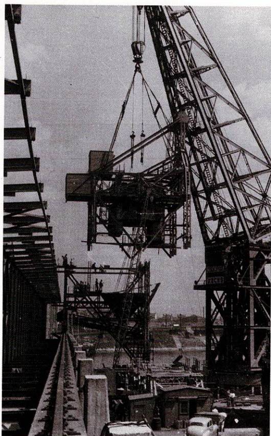
Above Erecting bulk raw sugar unloading cranes, 1955
