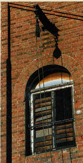
Materials access to the top of the cistern head.
