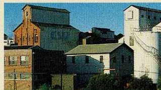
A south western view of the plant incorporating part of Hopkins Hall, the cistern house, bulk store, boiler station and oil tank.
