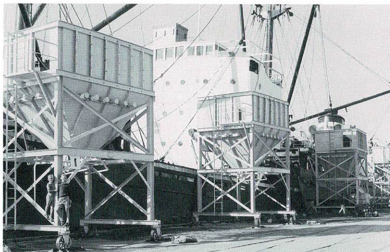
Huge hoppers in place after the change to bulk handling at Refinery Wharf.
