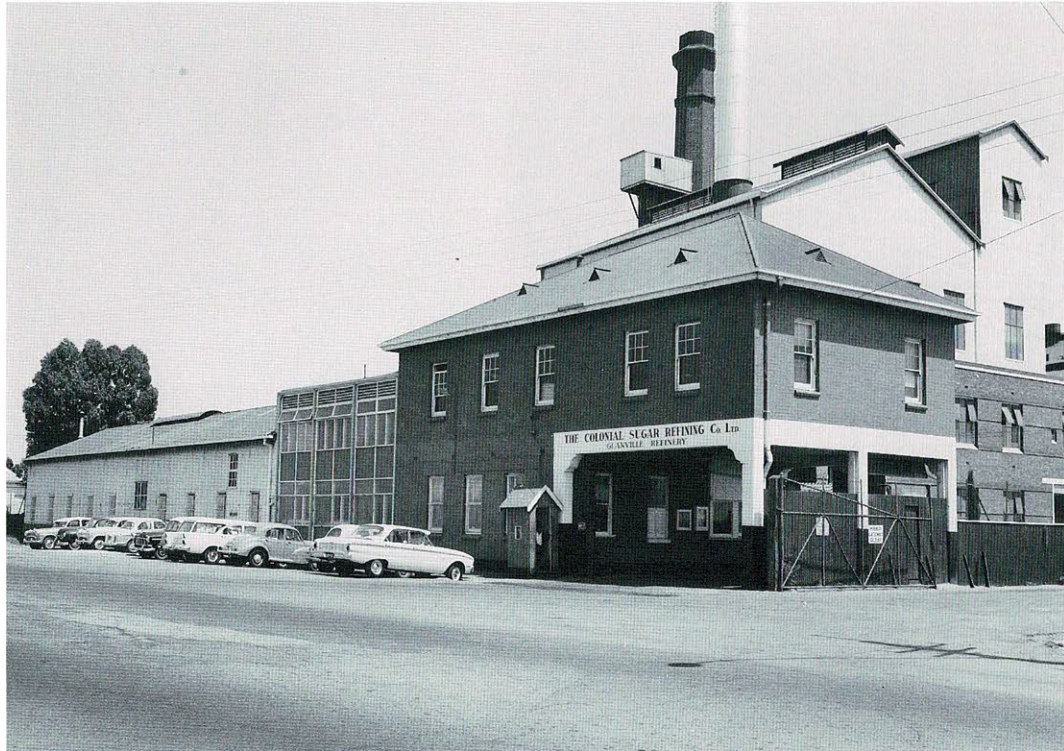
The refinery in the 1950s. A significant upgrade vastly improved its appearance.
