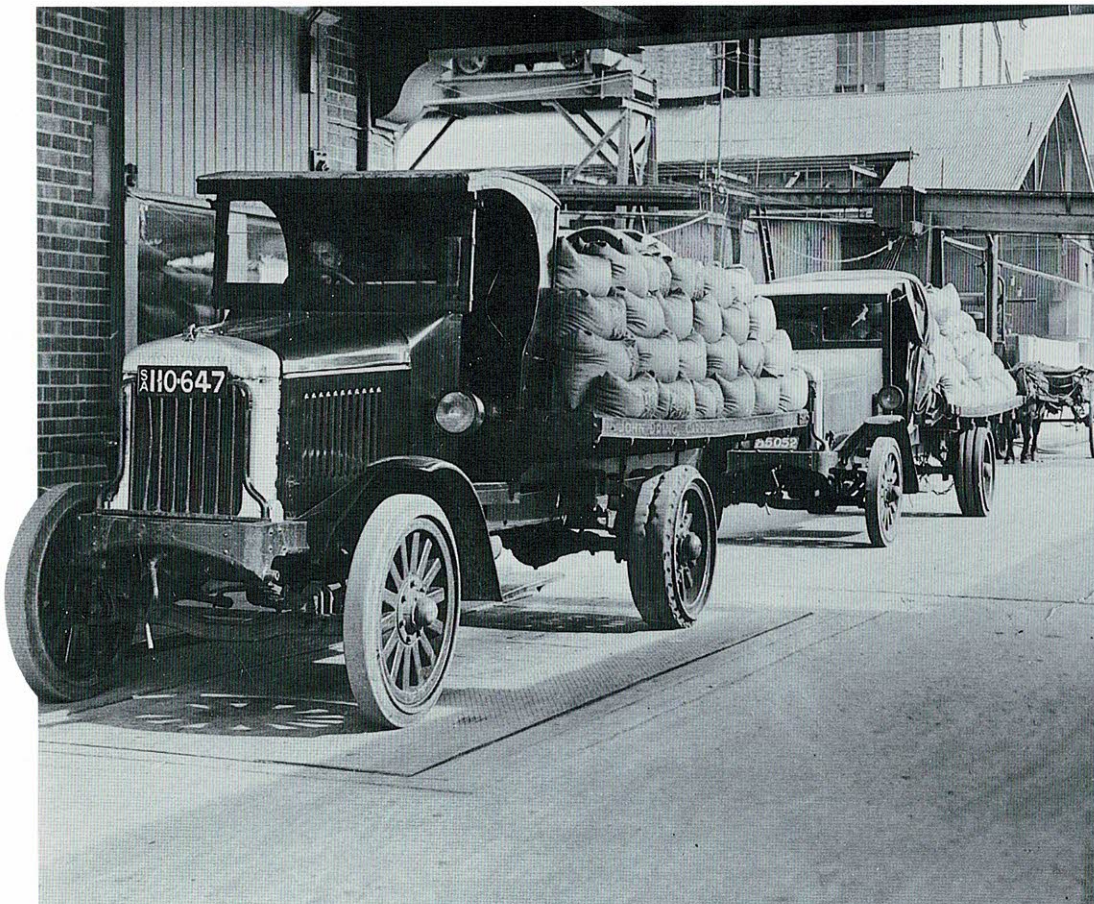
The plant's beam weighbridge. Don Bull recalls the problems horses pulling trolleys faced because of the two steel plates visible on each side of the weighbridge : "Because of their steel shoes, the horses would slip on the steel plates and fall head over heels. They'd have to get the horses up before they could go on."
