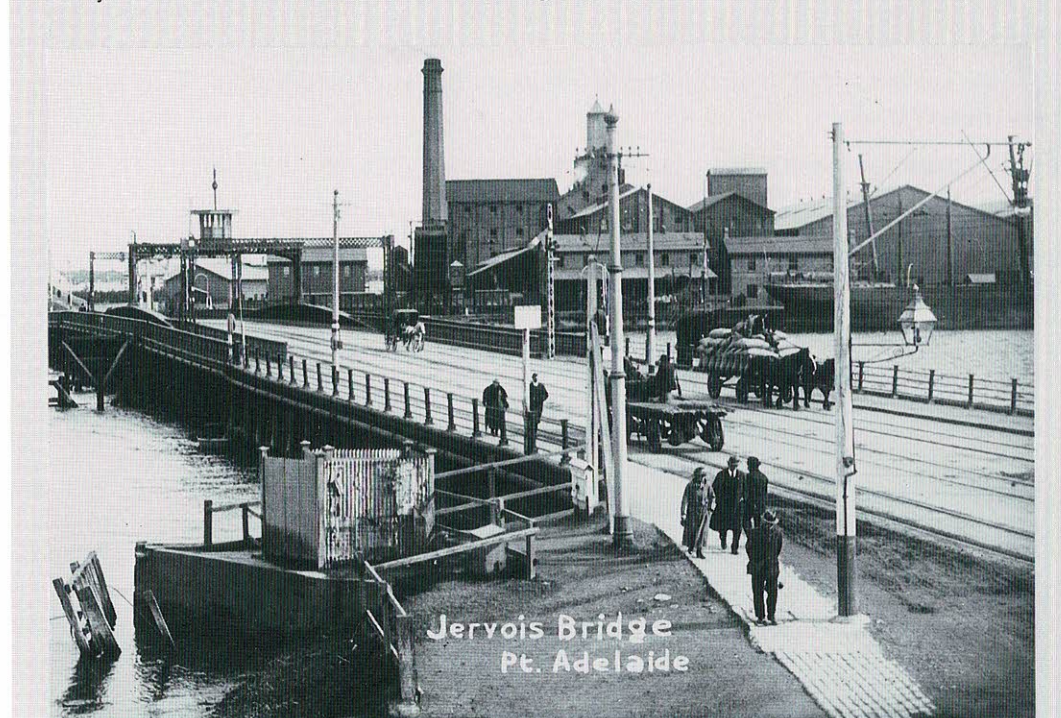
By 1919 the plant, with impressive smoke stack, dominated the scene looking across the Jervois Bridge and the Port River. Entrance to the plant was gained through an archway in the brick building on the right.
