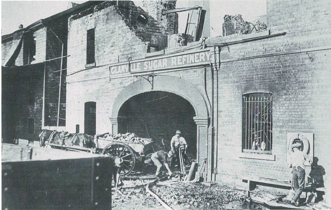
The factory entrance after the blaze.
