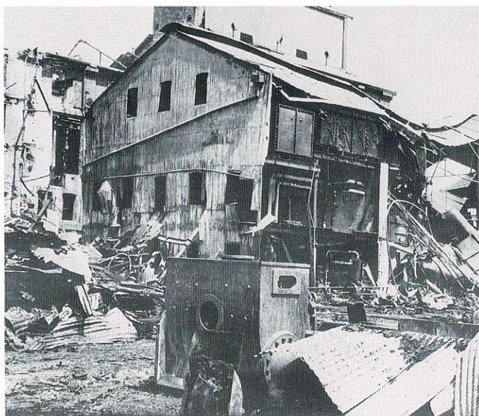
The devastation caused to the pan house and tank house viewed from the Port River.
