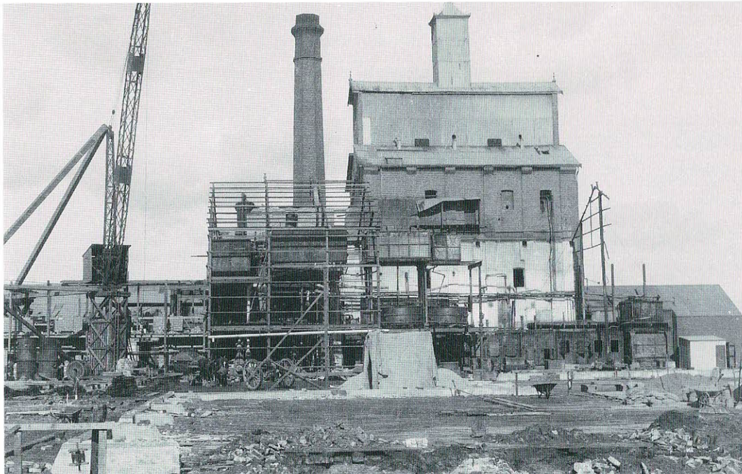
The rebuilding process began immediately after the fire. A crane lifts sections of the new plant framework.
