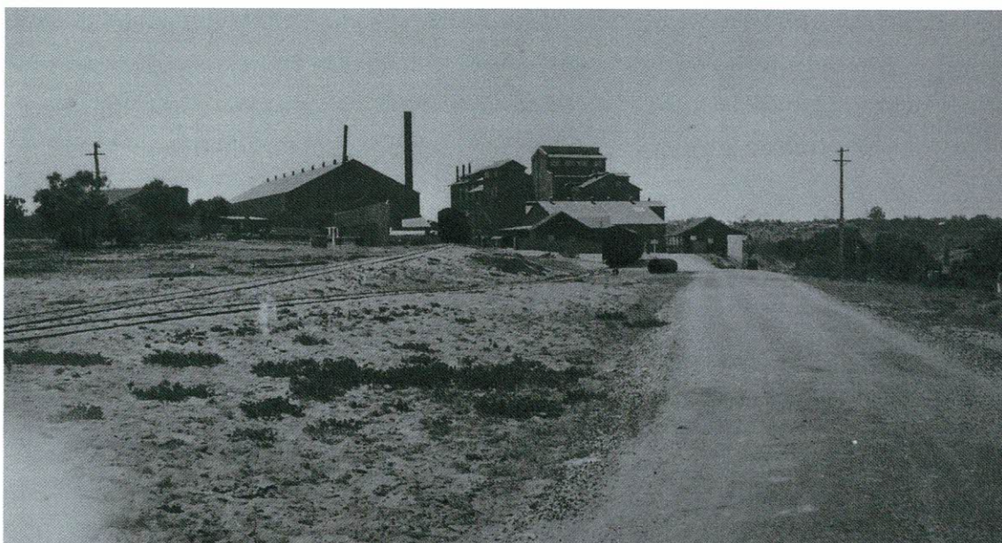
The refinery entrance in 1930. Note the railway track. The left-hand line was used to transport raw sugar to the raw sugar store; the line on the right carried packaged refined sugar away from the plant.
