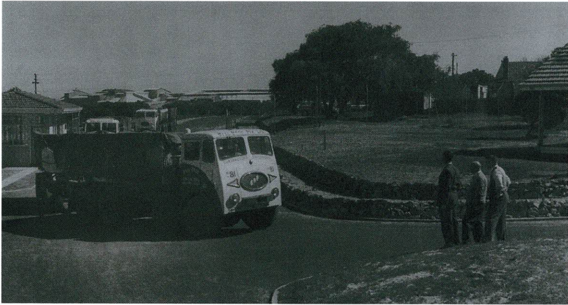
Convoy of raw sugar trucks arrive at the refinery. The old canteen can be seen far right.
