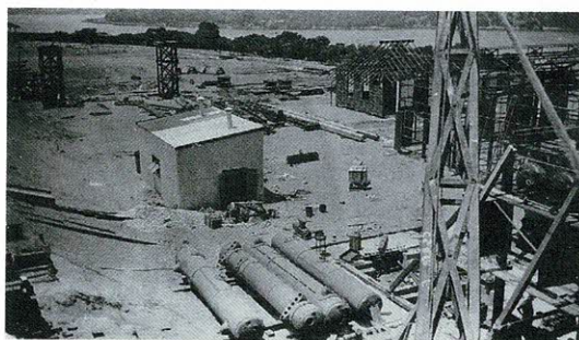
Construction, 1928 - 1930. Boiler drums (foreground) lie ready to be installed.
