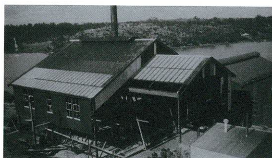
Construction, 1928 - 1930. The completed boiler station, with the char end under way.
